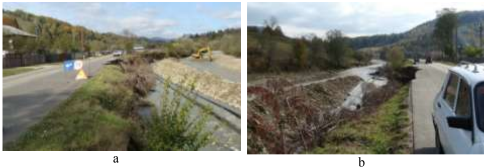
Fig. 5. The degradation phenomena of the riverbed in Zone 3, "Chiosa" after the flood in June 2016 on the Tazlăul Sărat River: a - upstream view of the river bed change and erosion; b - downstream view, highlighting oil piping and breaking the DC180A (photo Oct 2016)
