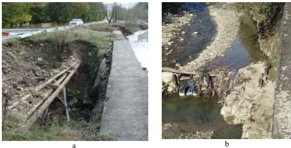
Fig. 7. Erosion phenomenon of the left bank after the flood in June 2016 on the Tazlăul Sărat River in Zone 4 "Forest Canton of Maxim": a - general view of the erosion zone behind the shore defence at the DC 180A limit; b - fencing phenomenon in the shore defence foundation area (Oct. 2016)
