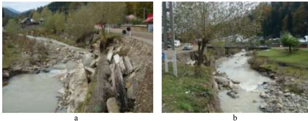
Fig. 4. General view of the morphology of the Tazlăul Sărat riverbed and the state of degradation of shore defence and DC 180A in Zone 1 "Toderaş": a - general view from downstream with highlighting the erosion of the road; b - upstream view (Oct 2016)
